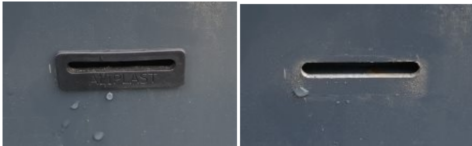
Operable and Fixed Panel Glazing Cavity Drainage
