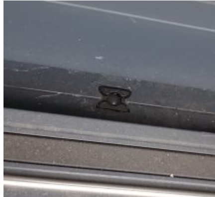
Operable Track Drainage with Check Ball Valve Insert
