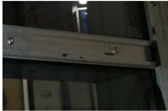
Drain slot in the pressure plate
