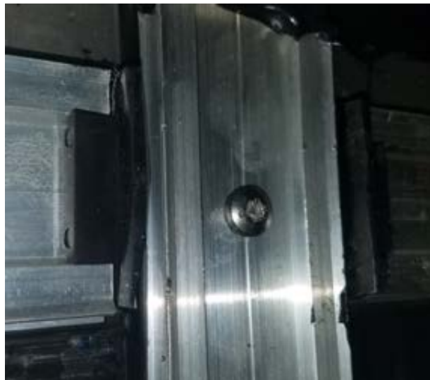
Pressure plate junction between horizontal and vertical
