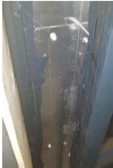
Install flashing on the interior
