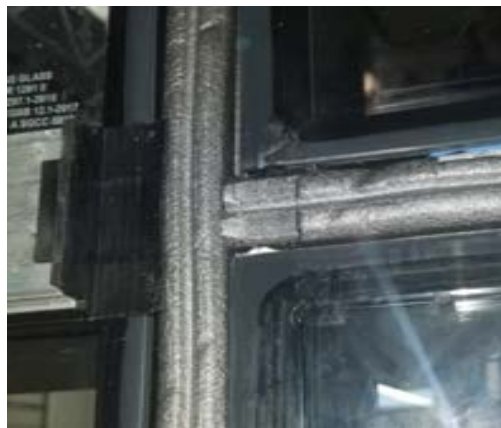
Foam used around the sealed units
