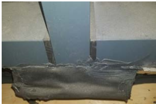
Installation bracket covered with fabric membrane
