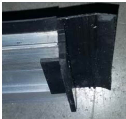
Pressure plate end dam gasket
