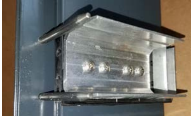
2x aluminum shear blocks and 2x stainless steel dowels
