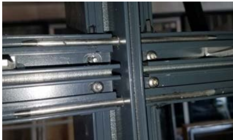
Vertical mullion to horizontal mullion joints
