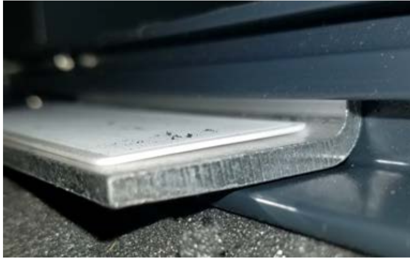
Setting block and aluminum carrier
