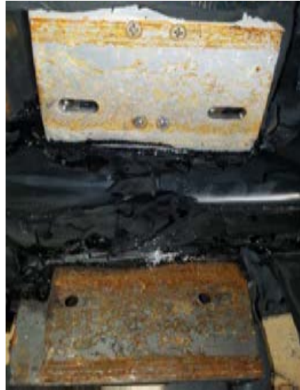
Installation bracket and aluminum plate attached to mullion bottom
