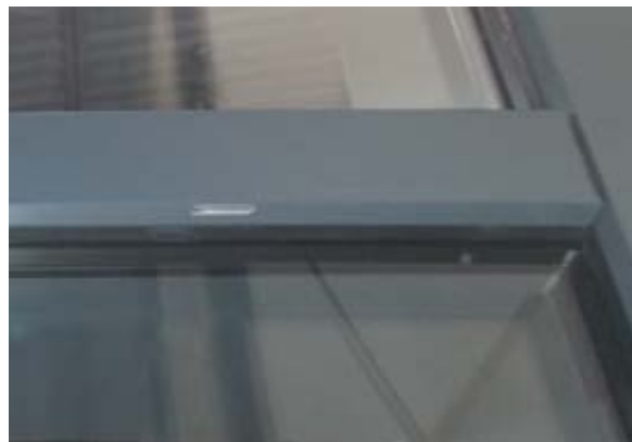
Drain slot in the pressure plate beauty cap
