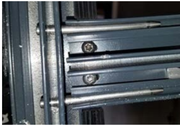
Jamb to horizontal mullion corner joint
