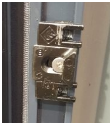
Multi-Point Lock Keeper
